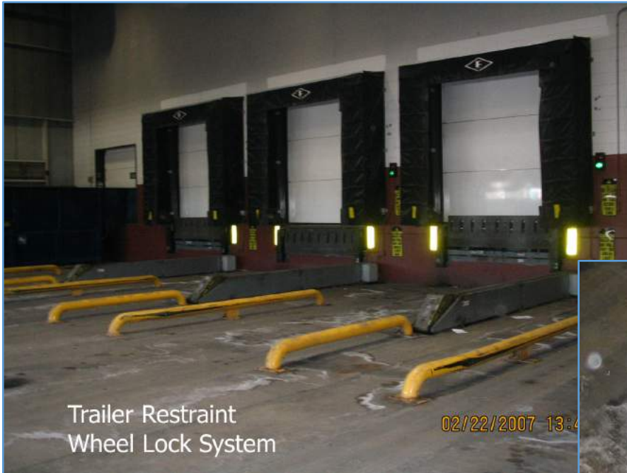
Trailer Restraint Wheel Lock Secures Trailer
